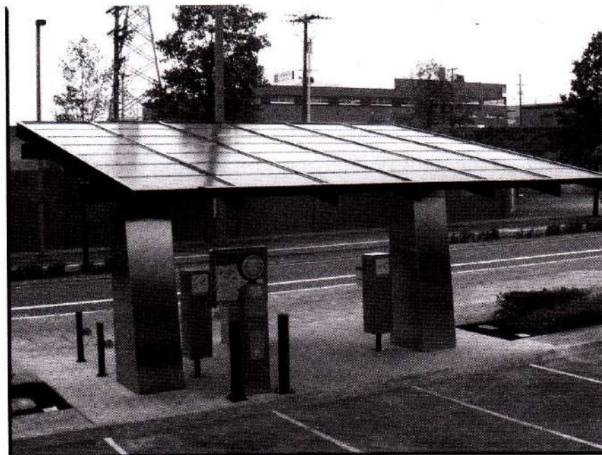
Figure 4. Solar PV charging station
